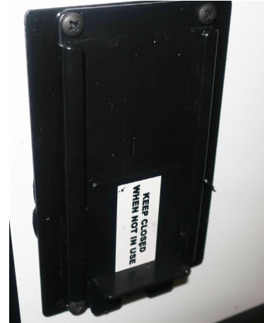
Cable QuickPort® (Located in the gear garage). -Typical View
